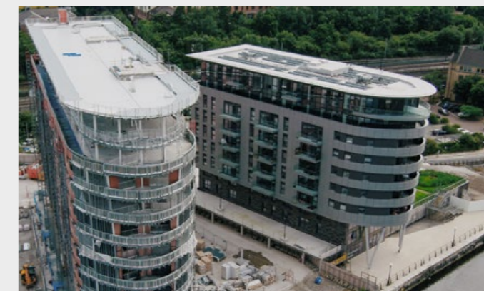
Drone image of the completed Tower A and Tower B which is under construction
