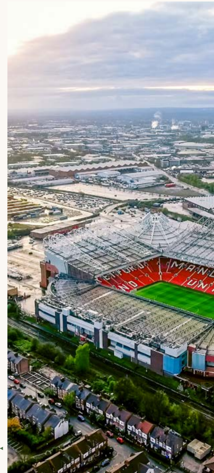
Old Trafford Stadium ◀
